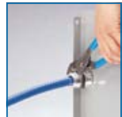
Hand tighten gland nut to hold cable, then wrench tighten
