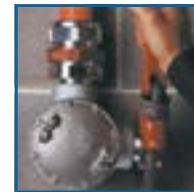
5. Install hub on enclosure
