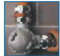
6. Insert cable and tighten red union
