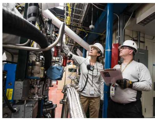
The stainless steel wire braid minimizes volumetric expansion in hydraulic service.
