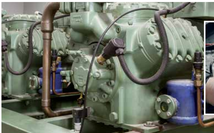
Presetting or adjustment of the pressure switch of a compressor
